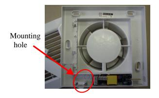
2. Connect the fan with power supply using the terminal strip on electronics. Usually goes from wall electric cable with 3 wires, so the blue is directly earthed conductor (N), brown / black is the phase conductor (L – under constant voltage) and third yellow-green is the circuit protective conductor (no need to connect when mounting plastic fan, can be blinded).
