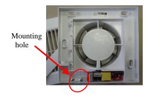
2. Connect the fan with power supply using the terminal strip on electronics. Usually goes from wall electric cable with 3 wires, so the blue is directly earthed conductor (N), brown / black is the phase conductor (L – under constant voltage) and third yellow-green is the circuit protective conductor (no need to connect when mounting plastic fan, can be blinded).
